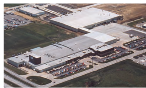
AGM Battery Manufacturing Plant, Warrensburg, MO, USA
